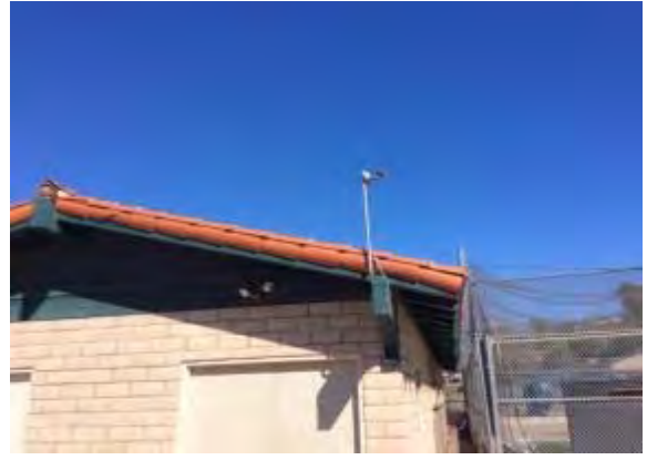
Photo #8: Partial view roofing
