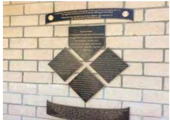
Photo #10: Exterior veneer brick wall
