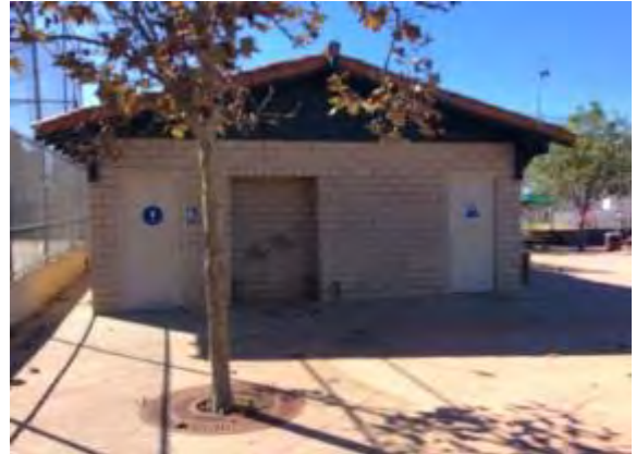
Photo #4: Side view of main building
