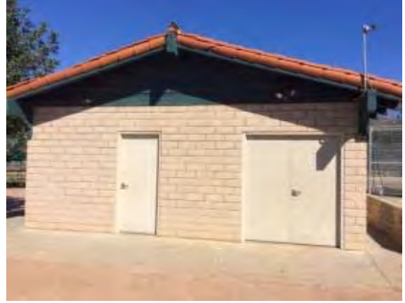
Photo #2: Side view of main building
