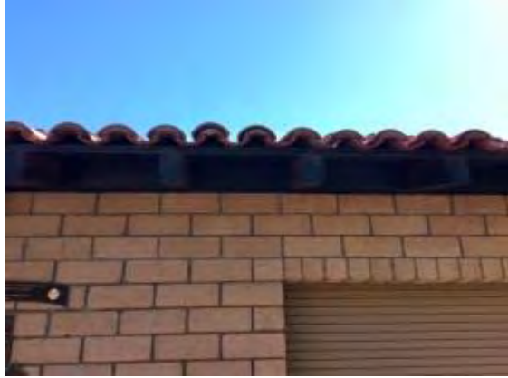
Photo #7: Partial view of roofing
