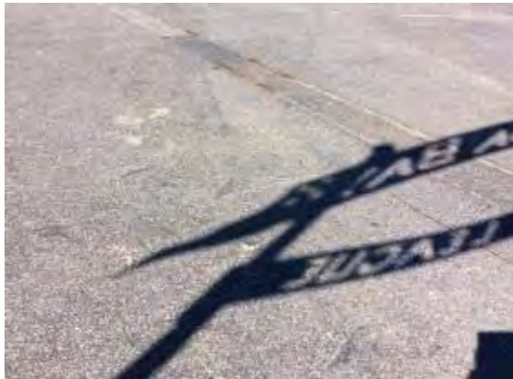
Photo #5: Asphalt pavement
