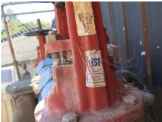
Photo #29: Water service backflow device
