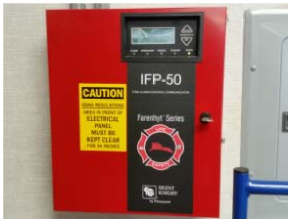
Photo #41: Fire alarm panel
