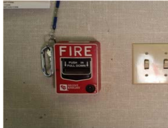
Photo #40: Fire alarm pull station
