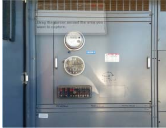
Photo #26: Main 2000 amp electrical service
