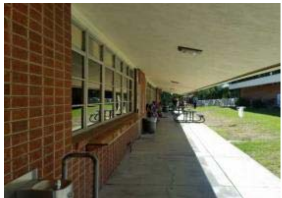
Photo #18: Enclosed soffit
