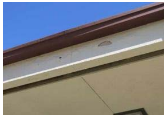
Photo #54: Paint spalling
