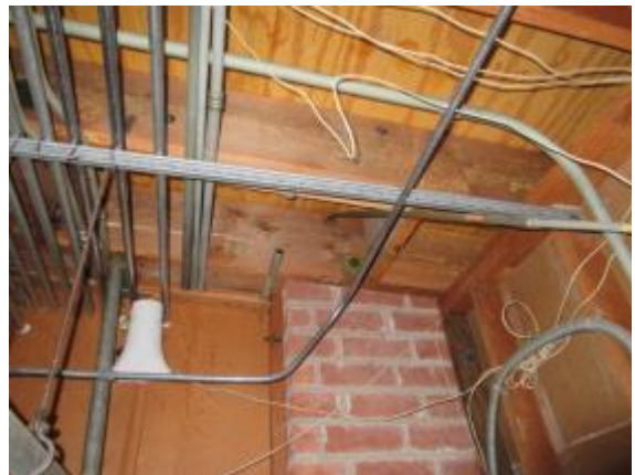
Photo #16: Roof structure
