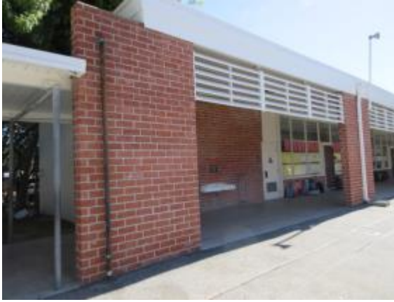
Photo #19: Overhang structure
