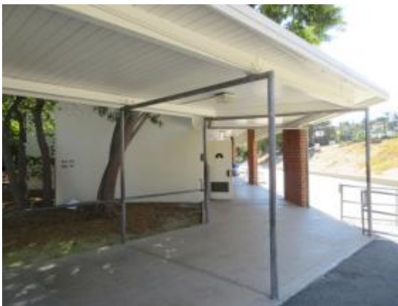
Photo #23: Walkway shade structure
