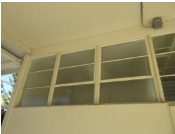
Photo #17: Classroom windows
