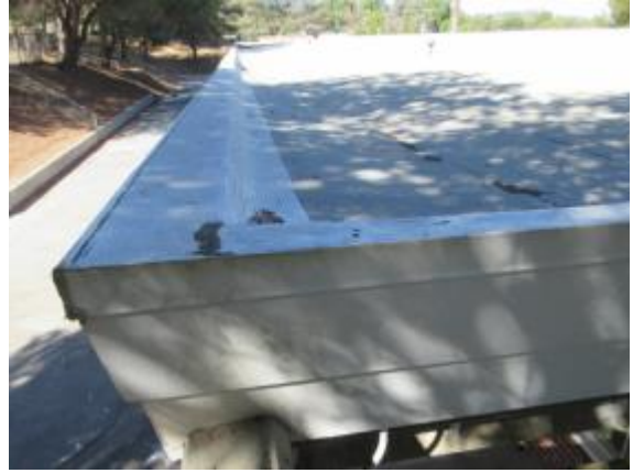
Photo #14: Roof flashing
