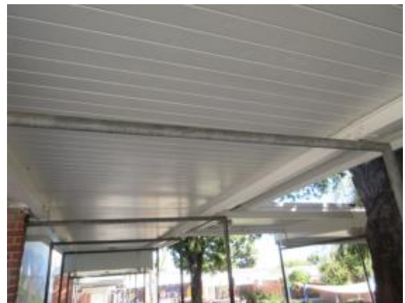
Photo #24: Walkway shade structure
