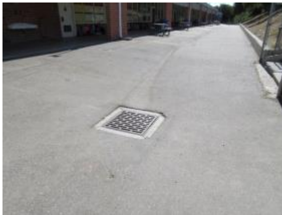
Photo #9: Storm drain
