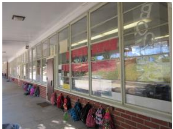
Photo #18: Classroom windows
