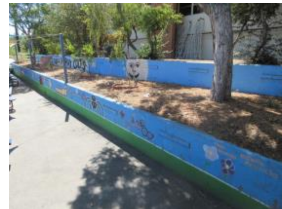
Photo #12: Retaining walls
