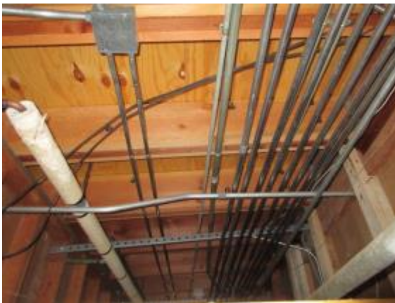
Photo #15: Roof structure
