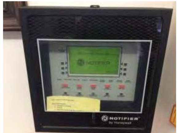
Photo #42: Fire alarm control panel
