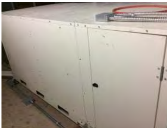
Photo #41: Above ceiling fan coil unit
