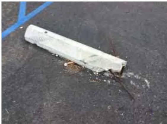
Photo #15: Damaged wheel stop at lower parking lot
