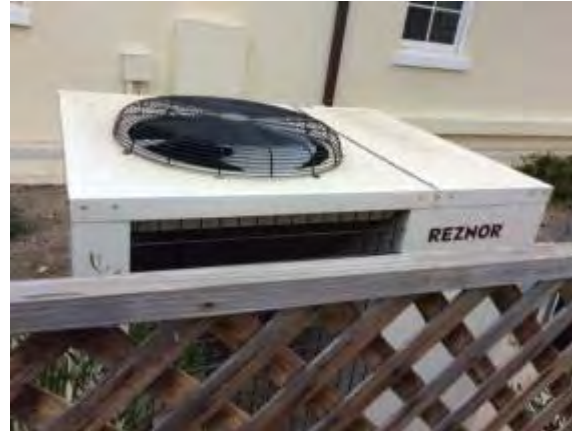
Photo #50: Condensing unit
