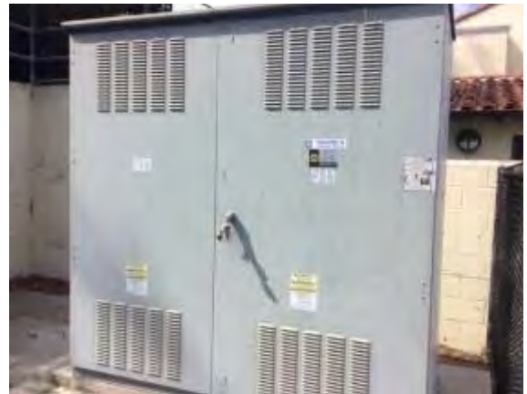
Photo #46: Main electrical switchgear
