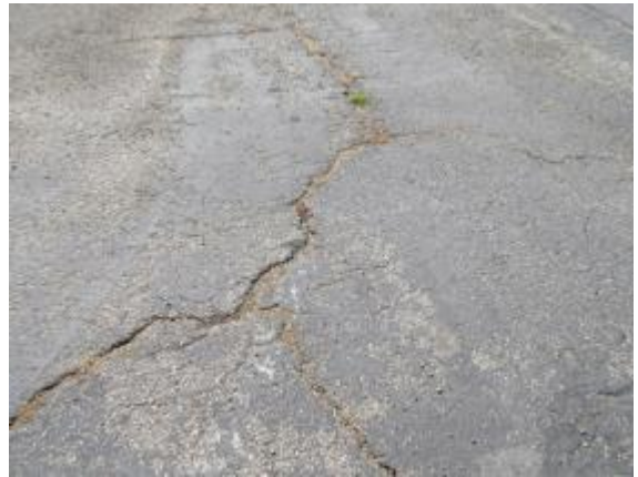
Photo #58: Basketball/volleyball court asphalt in poor condition
