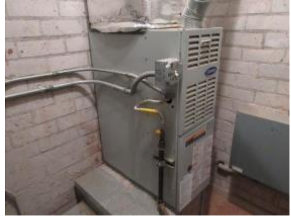
Photo #38: Forced-air furnace
