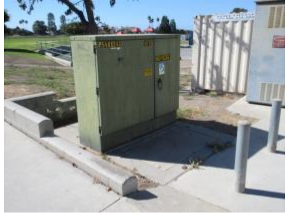
Photo #32: Main transformer
