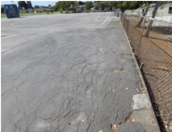
Photo #57: Playground asphalt in poor condition
