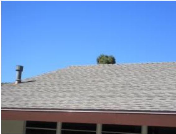
Photo #20: Asphalt shingle roof
