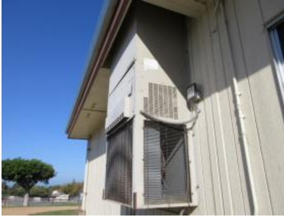
Photo #37: Package heat pump
