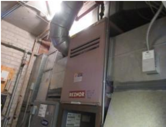
Photo #39: Duct furnace
