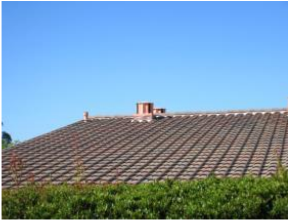
Photo #19: Clay tile roof
