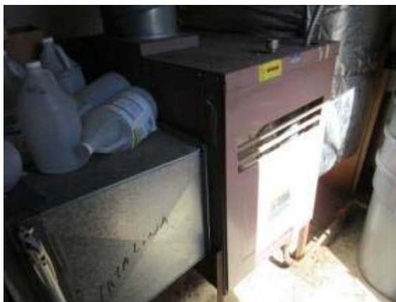
Photo #23: Duct furnace
