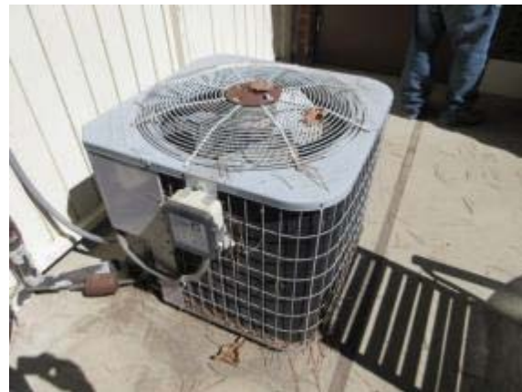
Photo #22: Split AC condensing unit
