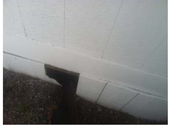
Photo #38: Deteriorated wood siding
