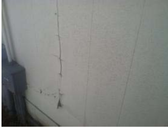
Photo #37: Deteriorated wood siding
