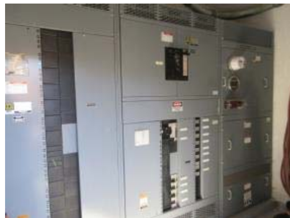
Photo #24: Electrical switchgear
