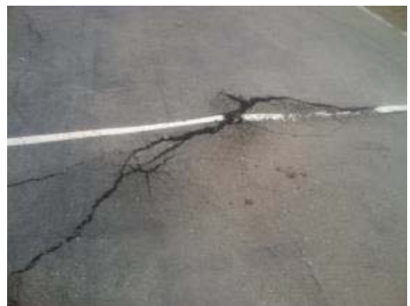
Photo #42: Damaged basketball court asphalt
