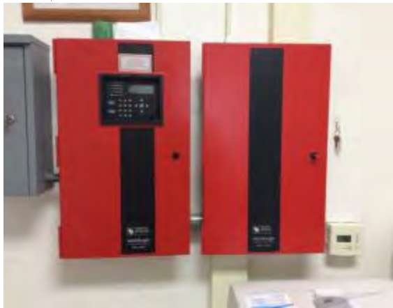
Photo #21: Fire alarm control panels
