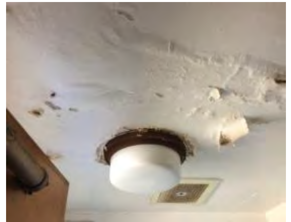
Photo #40: Fungal growth (unused restroom at MPR)
