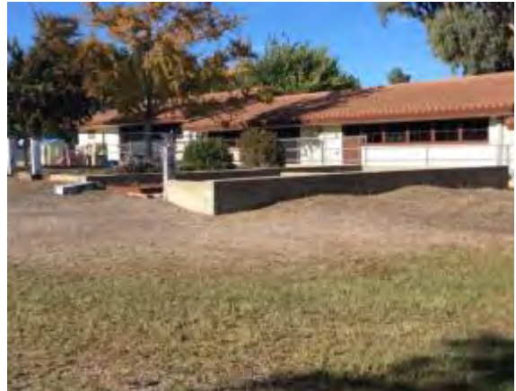
Photo #16: Clay tile roof
