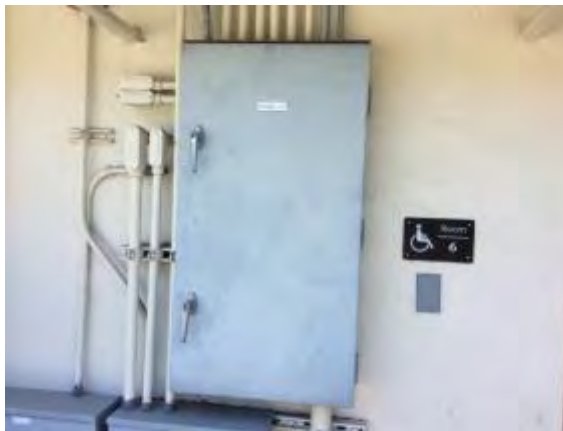
Photo #29: Circuit breaker panel
