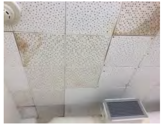
Photo #34: Acoustical ceiling tiles (glued)
