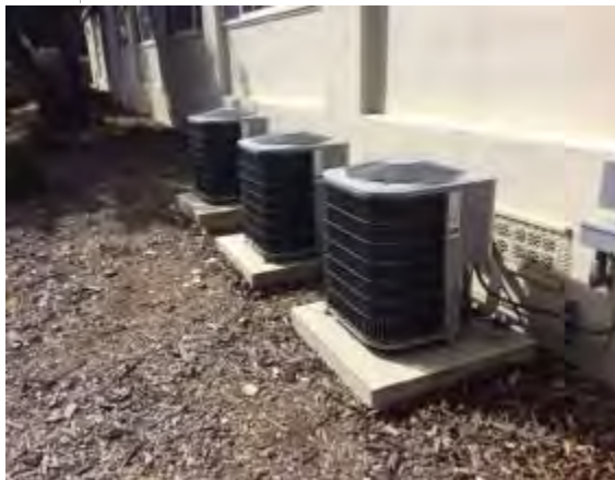
Photo #23: Condensing units
