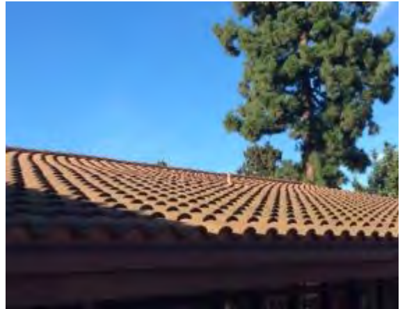
Photo #14: Clay tile roof
