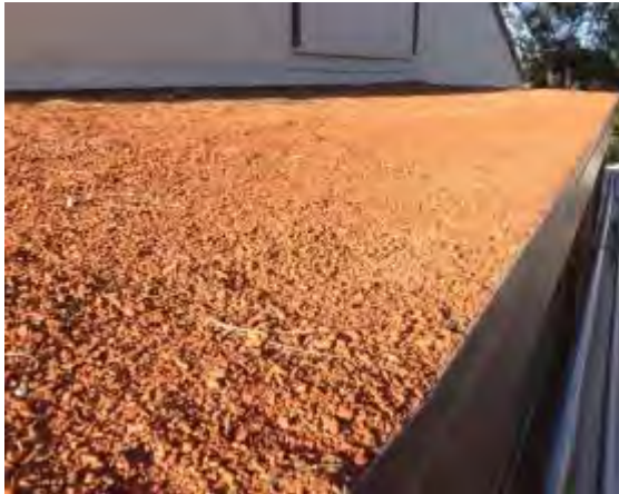
Photo #13: Built-up roof at covered walkway
