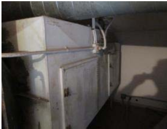
Photo #21: Duct heater
