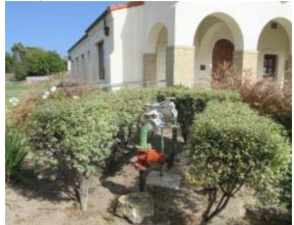
Photo #28: Backflow device
