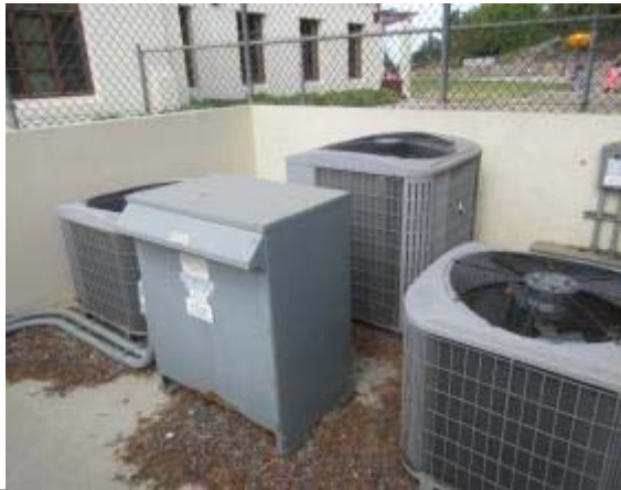
Photo #19: HVAC condensing units and transformer
