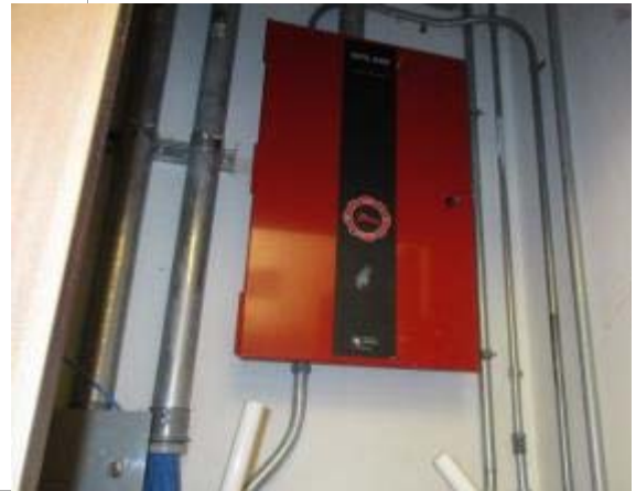
Photo #36: Fire alarm panel
