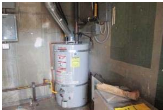
PHOTO #42: WATER HEATER, GAS, RESIDENTIAL, 30 TO 50 GAL
