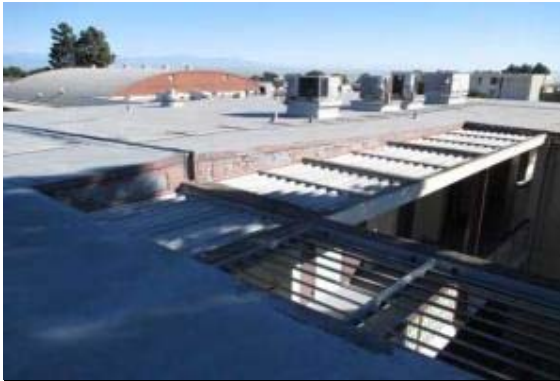
PHOTO #25: ROOF, MODIFIED BITUMINOUS
