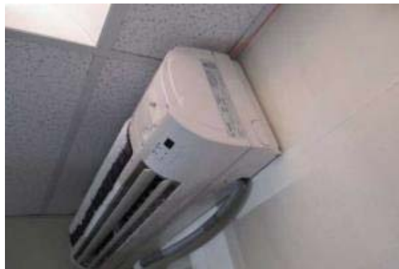
PHOTO #34: DUCTLESS SPLIT SYSTEM, SINGLE ZONE, 0.75 TO 1 TON
