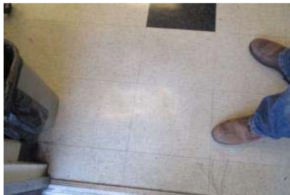
PHOTO #48: INTERIOR FLOOR FINISH, VINYL TILE (VCT)
