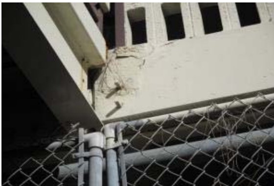
PHOTO #15: STEEL SUPPORT AT SECOND STORY WALKWAY IS RUSTING AND CAUSING SPALLING
