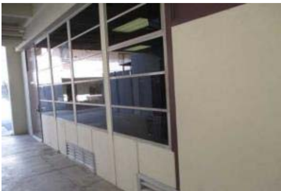
PHOTO #29: WINDOW, ALUMINUM DOUBLE-GLAZED 24 SF, 1-2 STORIES
