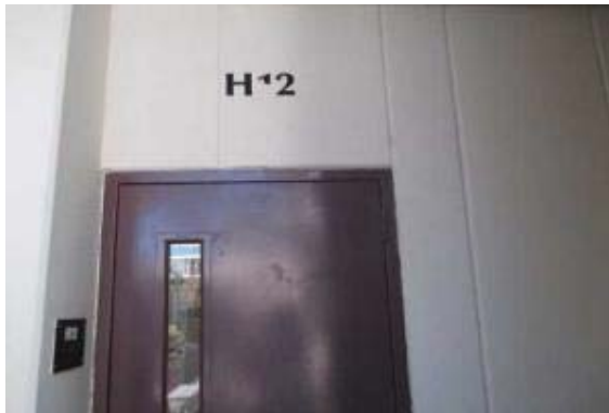
PHOTO #31: EXTERIOR DOOR, STEEL WITH SAFETY GLASS
