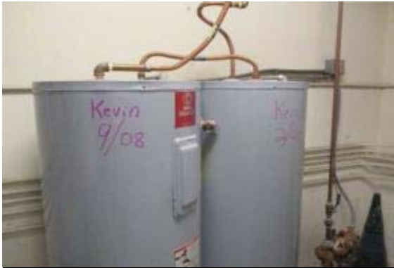
PHOTO #43: WATER HEATER, ELECTRIC, COMMERCIAL, 30 TO 80 GAL
