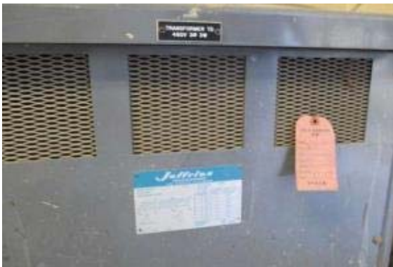
PHOTO #45: SECONDARY TRANSFORMER, DRY, 113 KVA
