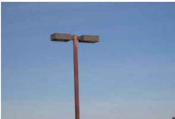
PHOTO #23: METAL HALIDE LIGHTING FIXTURE, 250 W
