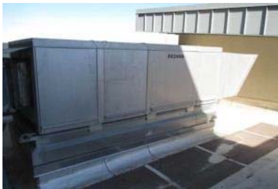
PHOTO #35: MAKE-UP AIR UNIT, 6,001 TO 12,000 CFM
