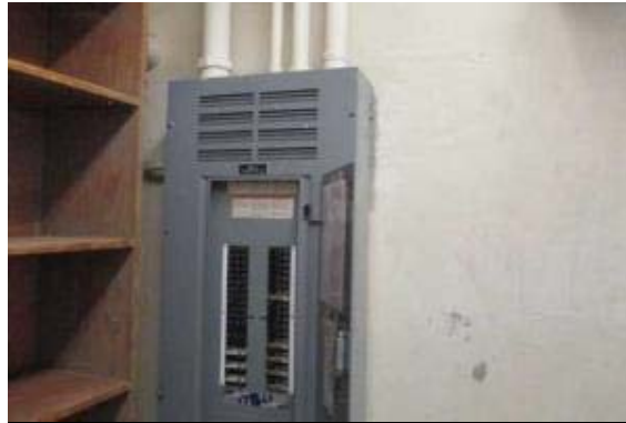
PHOTO #44: DISTRIBUTION PANEL, 208 Y, 120 V, 225 AMP
