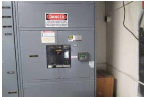
PHOTO #46: BUILDING/MAIN SWITCHGEAR, 480 Y, 277 V, 2,000 AMP
