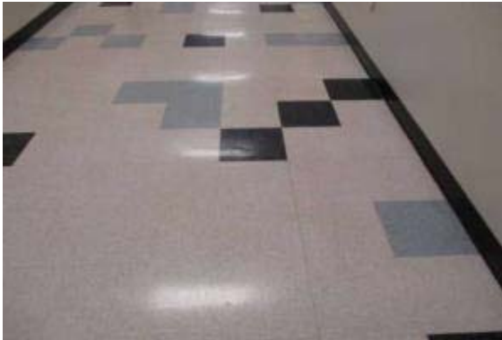
PHOTO #49: INTERIOR FLOOR FINISH, VINYL TILE (VCT)
