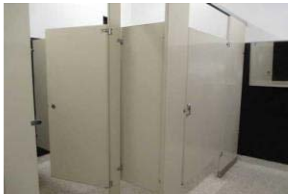
PHOTO #36: TOILET PARTITIONS, METAL OVERHEAD-BRACED
