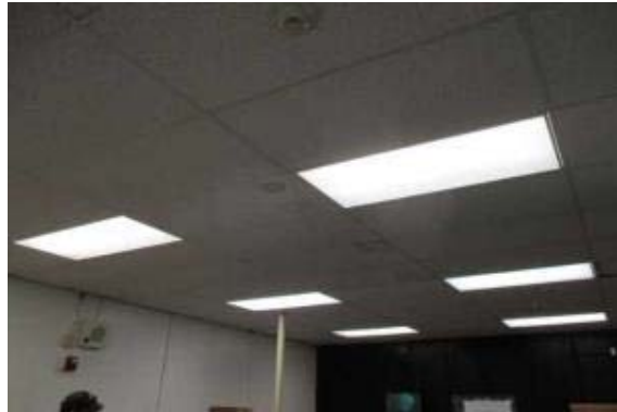
PHOTO #50: INTERIOR CEILING FINISH, ACOUSTICAL TILE (ACT)
