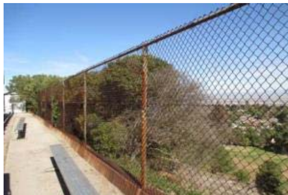
PHOTO #24: FENCES AND GATES, CHAIN LINK, 6' HIGH
