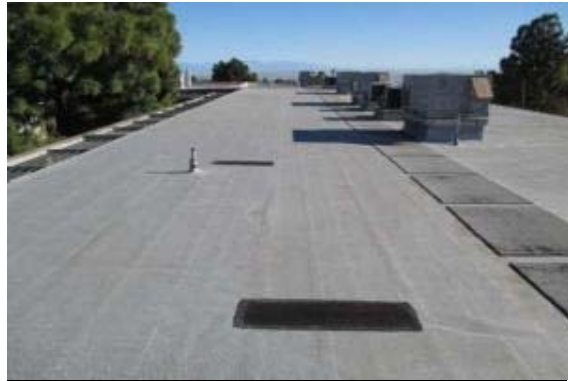
PHOTO #26: ROOF, MODIFIED BITUMINOUS
