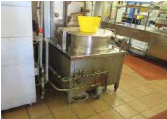
Photo #51: COMMERCIAL KITCHEN, STEAM KETTLE
