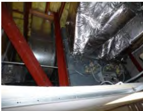
Photo #35: Air handler ceiling mounted and office building
