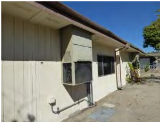
Photo #57: Wall mounted HVAC package units at portable buildings
