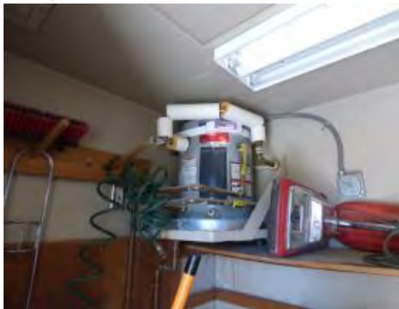
Photo #33: Hot water heater
