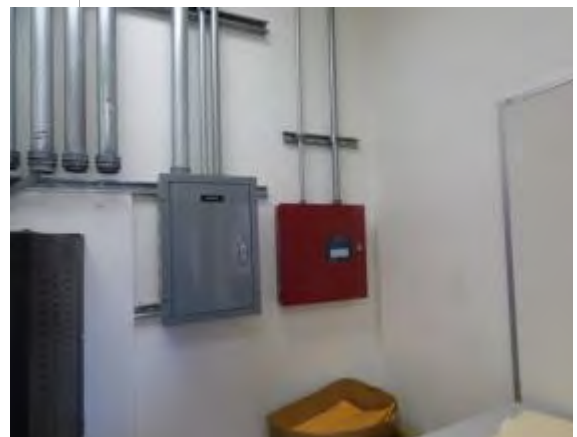
Photo #60: Fire Control Sub-Panels throughout all buildings
