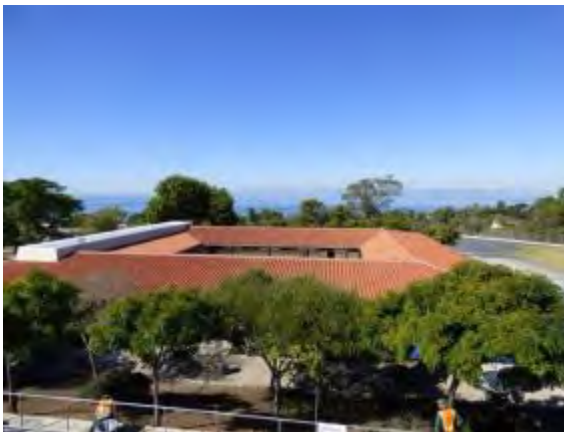
Photo #45: Concrete tile mansard roof overview
