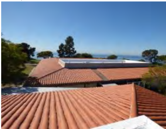
Photo #48: Concrete tile mansard roof overview
