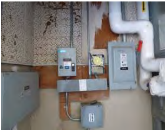
Photo #39: Air handler controls throughout classroom buildings
