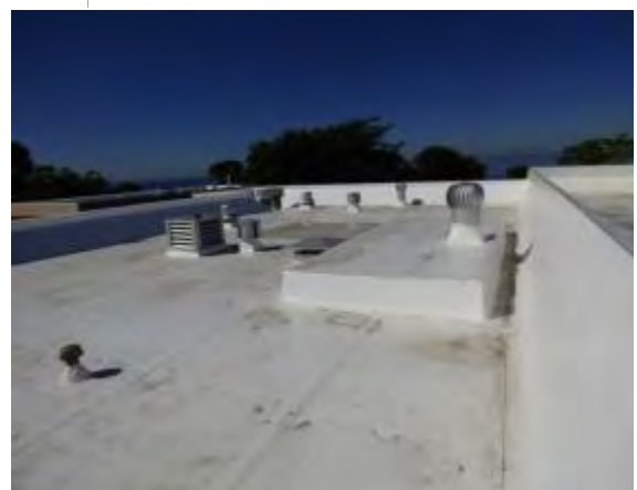
Photo #42: TPO single ply membrane roof
