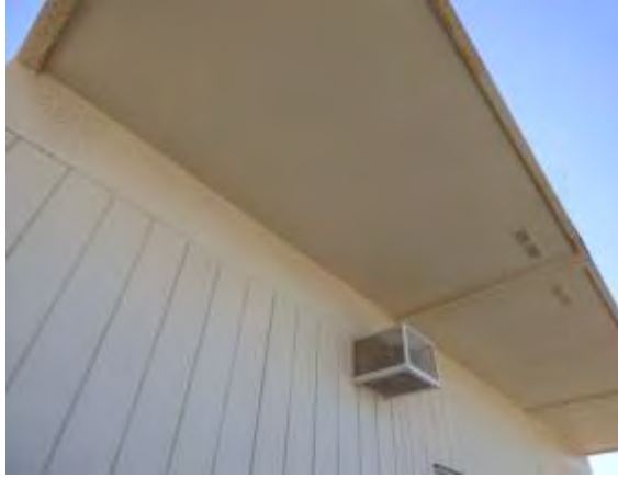
Photo #55: Soffit and exterior wall of portable buildings
