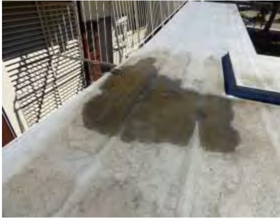
Photo #44: TPO single ply membrane roof (viewed at minor isolated ponding)
