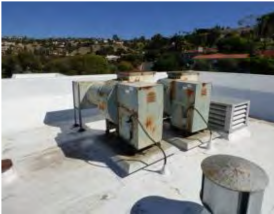
Photo #43: TPO single ply membrane roof (kitchen area vents)
