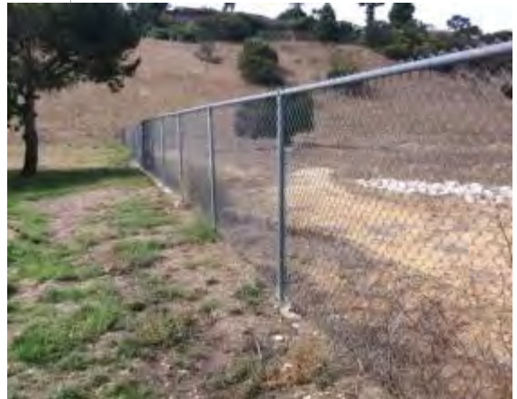
Photo #16: Chain link perimeter fence
