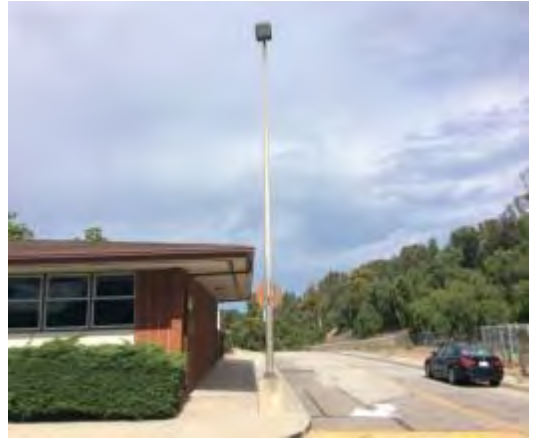
Photo #14: Site lighting
