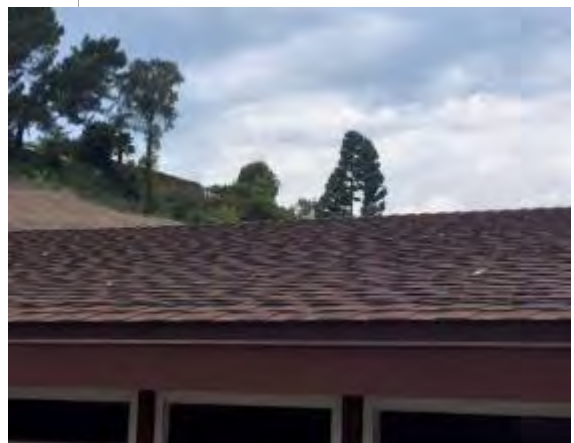
Photo #18: Asphalt shingles roof
