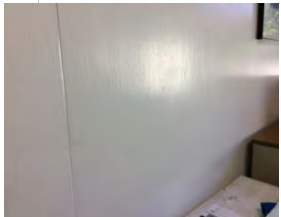
Photo #42: Painted Masonite panel interior wall
