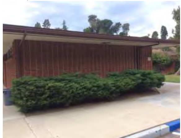
Photo #4: Side view of Classrooms Building
