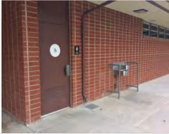
Photo #19: Masonry brick exterior wall
