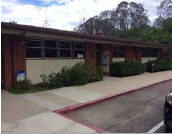
Photo #1: Front view of Administration Building
