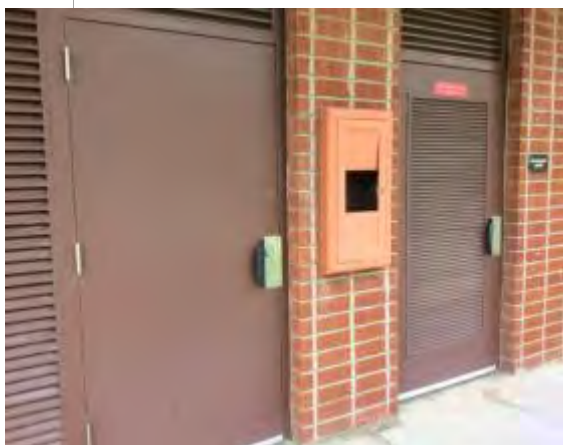
Photo #23: Exterior doors
