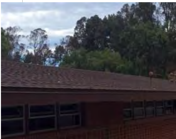
Photo #17: Asphalt shingles roof
