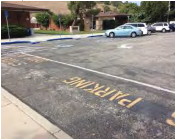
Photo #9: Parking lot with ADA parking spaces
