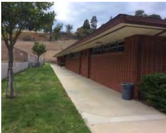
Photo #5: Rear view of Classrooms Building
