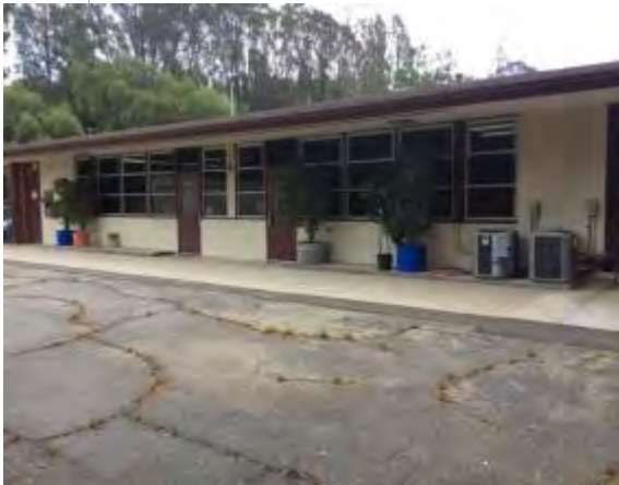
Photo #3: Rear view of Administration Building
