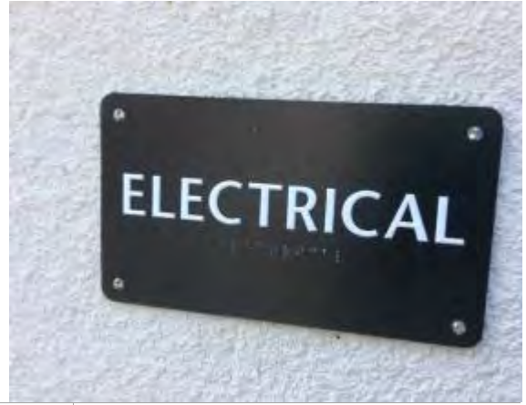
Photo #20: CMU exterior wall
