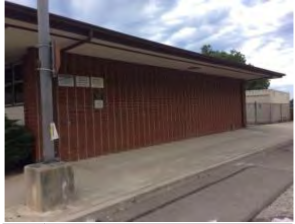
Photo #2: Side view of Administration Building
