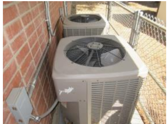
Photo #24: Classroom split Air Conditioner condensing units
