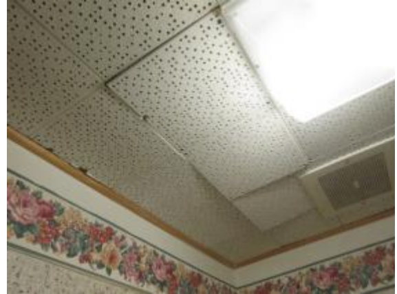
Photo #38: Damaged tiles at office ceiling
