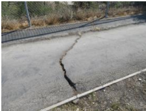
Photo #39: Damaged asphalt at east walkway
