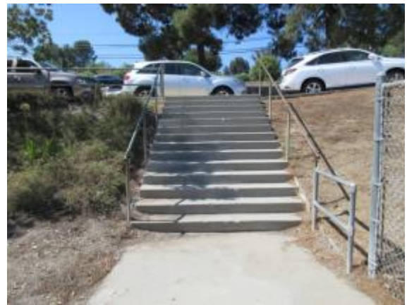
Photo #42: Handrails do not extend beyond stairs at northwest stairs
