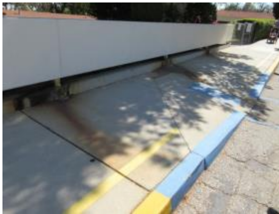
Photo #41: Rusty tube-steel supports at west entrance
