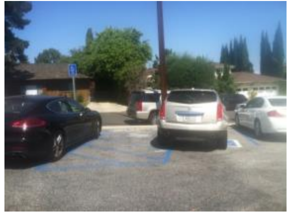
Photo #8: Missing sign at accessible parking space
