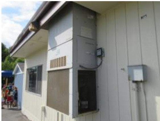
Photo #23: Modular classroom package heat pump
