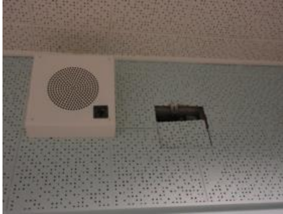
Photo #37: Damaged hard tile at office wall
