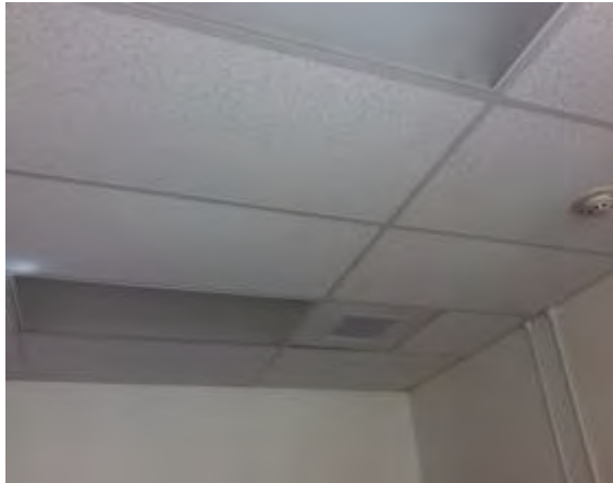
Photo #43: Suspended Acoustical Ceiling
