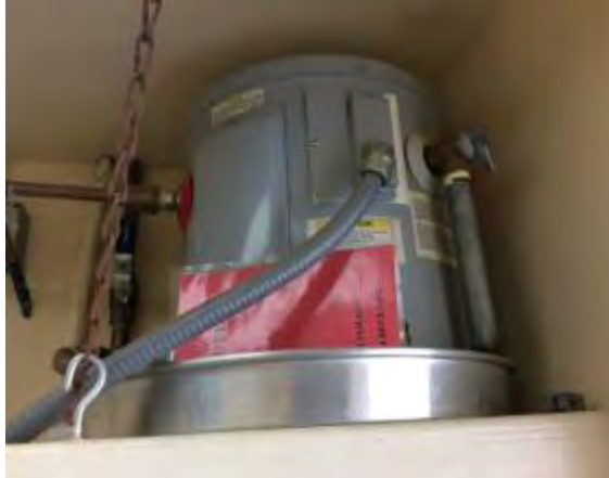
Photo #37: Electric Water Heater
