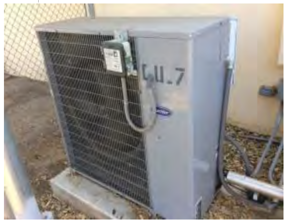
Photo #36: Condensing Unit
