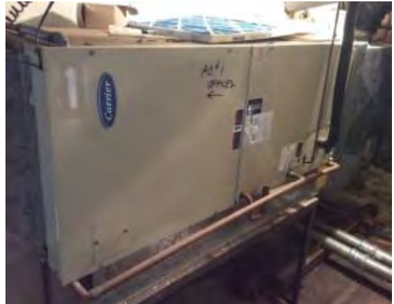
Photo #32: Fan Coil Unit
