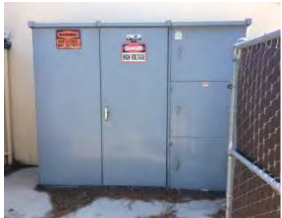
Photo #34: Main Switchgear
