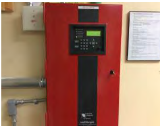
Photo #29: Fire Alarm Control Panel
