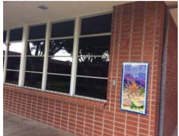
Photo #24: Aluminum-framed Operable Windows
