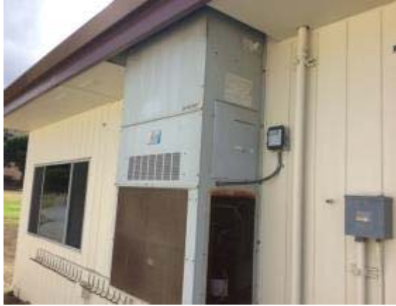
Photo #37: Wall-mounted Heat Pump
