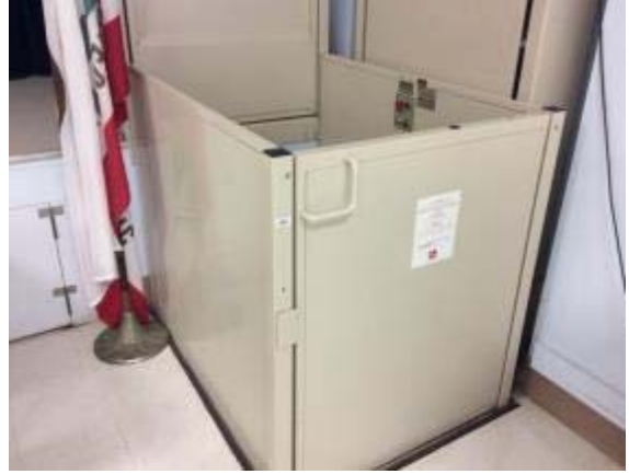
Photo #32: Wheelchair Lift
