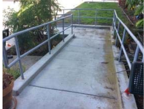
Photo #26: Concrete Ramp
