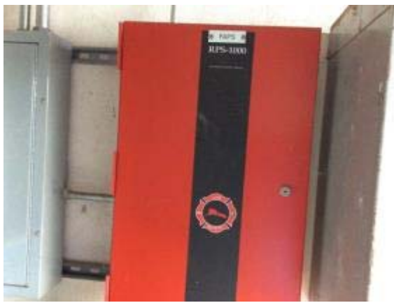
Photo #29: Fire Alarm Panel
