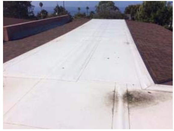
Photo #20: Asphalt Shingles w/PTO Roof
