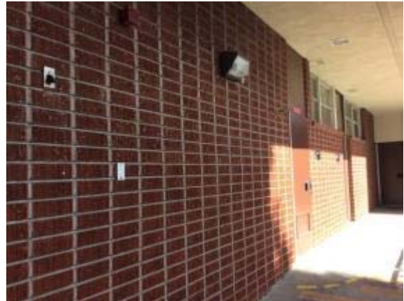
Photo #6: Side view of Building E
