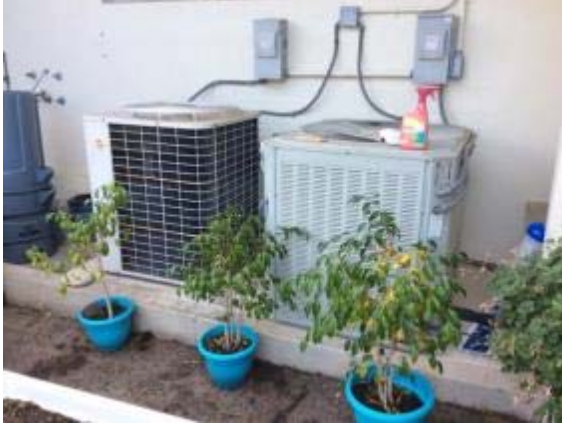
Photo #31: Pad-mounted Condensing Units
