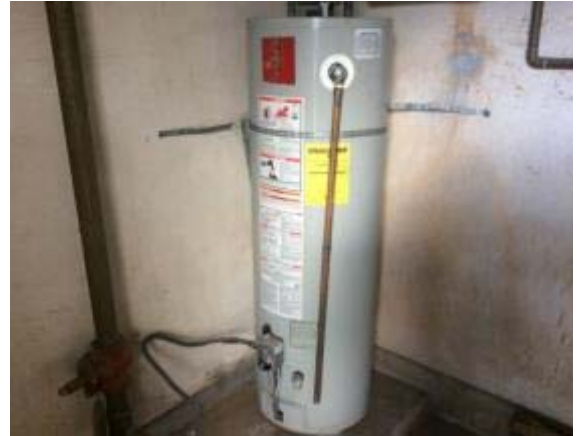
Photo #40: Water Heater
