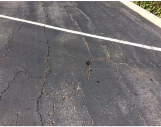
Photo #11: Asphalt roadway pavement
