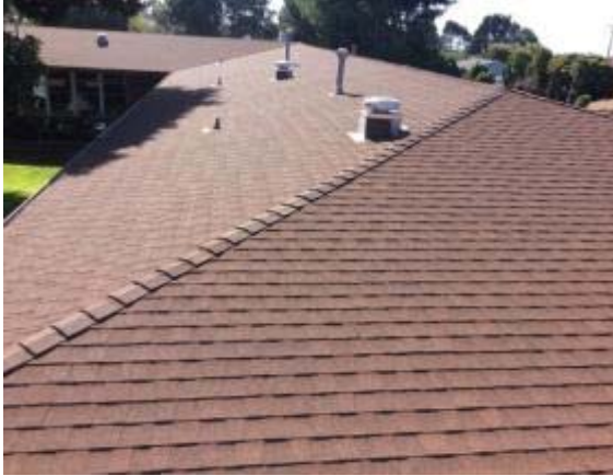
Photo #19: Asphalt Shingles Roof
