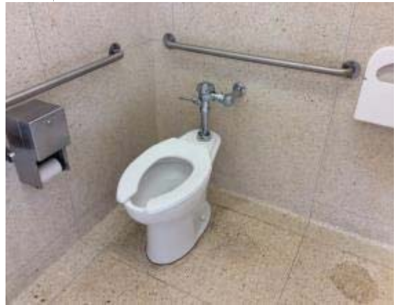
Photo #34: Water Closet
