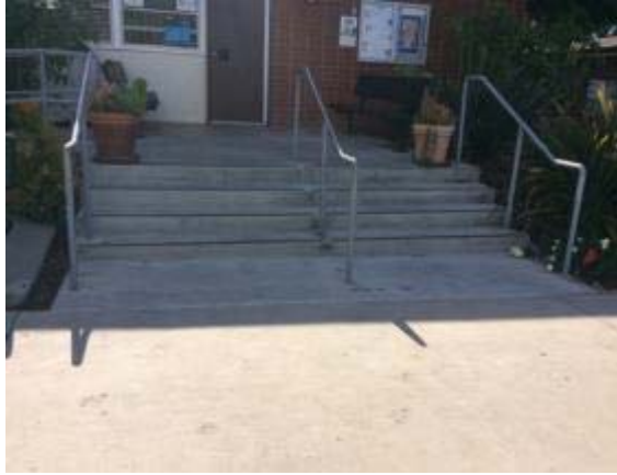
Photo #25: Concrete Exterior Stairs
