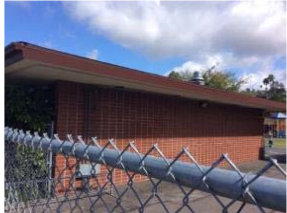
Photo #4: Side elevation of Kindergarten Building
