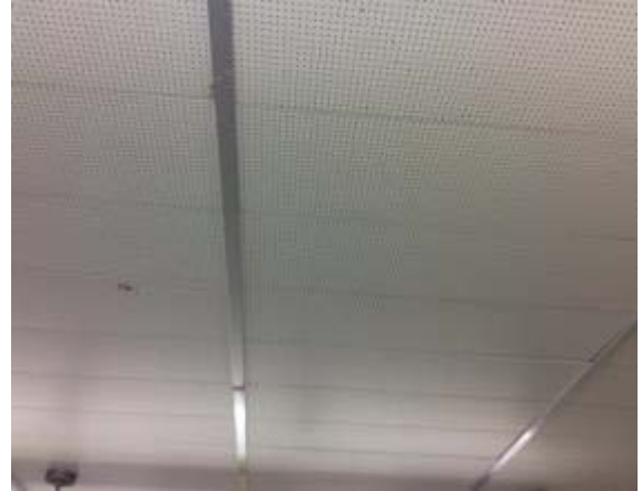
Photo #44: Glued Acoustical Ceiling Tiles
