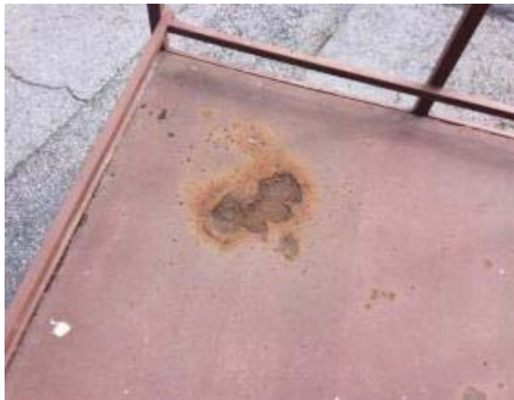
Photo #27: Metal Ramp
