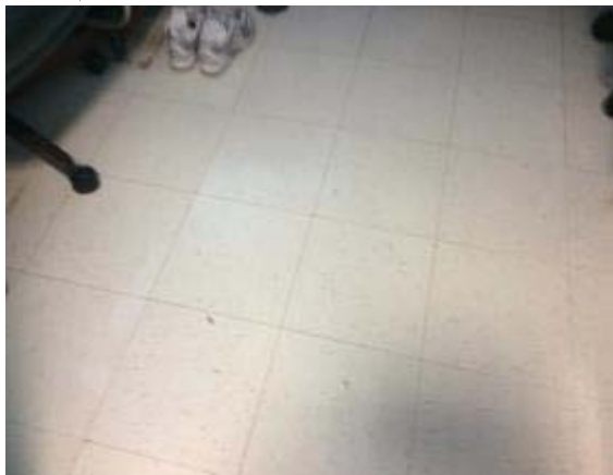
Photo #41: Vinyl Tile Flooring
