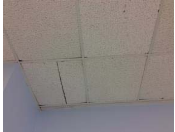
Photo #42: Acoustical Ceiling Tiles
