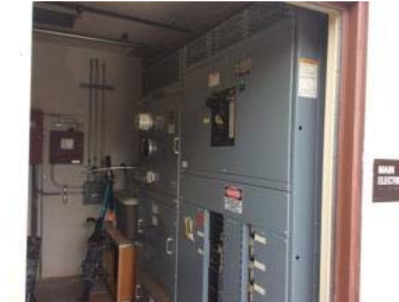
Photo #30: Main Switchgear
