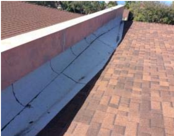
Photo #21: Parapet Wall
