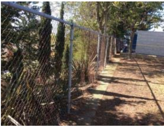
Photo #17: Chain link Perimeter Fence
