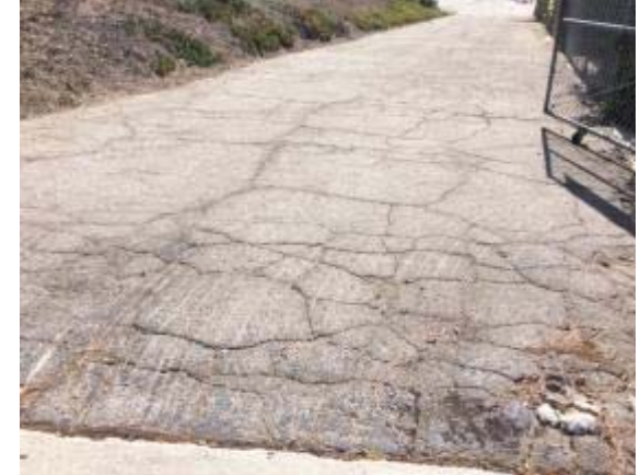
Photo #12: Asphalt roadway pavement
