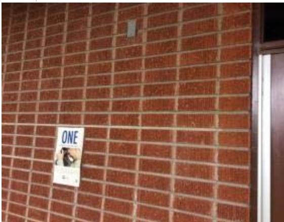
Photo #23: Veneer Exterior Wall
